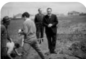
Laying foundations at Preca Centre, Ardeer 1960s.
